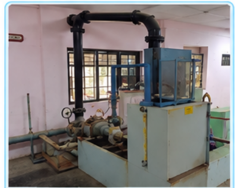
Centrifugal Pump Test
